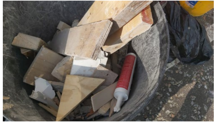
Figure 4: mixed waste arriving at the skip in a bin
