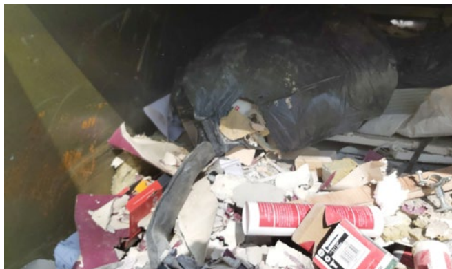
Figure 7: Boxes of screws, packaging & mixed demolition waste
