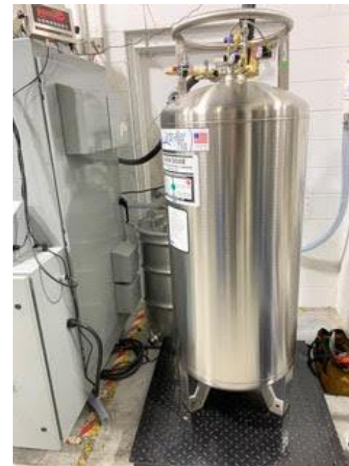
Dewar / Scale (33" W x 33" L x 68" H) Max Distance of Line -6'
