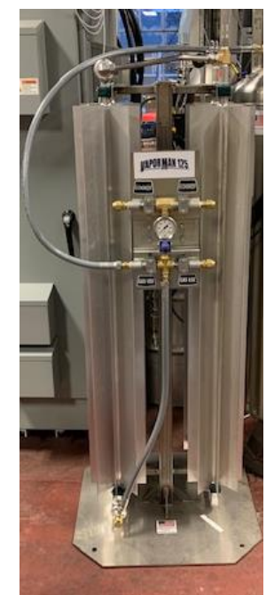
Vaporman (30" W x 30" L x 48" H) Max Distance of Line -6'
