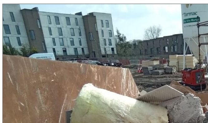
Figure 9: Plasterboard in mixed skip
