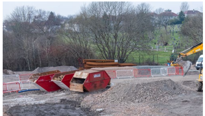
Figure 1: Skip compound on south side of the site
