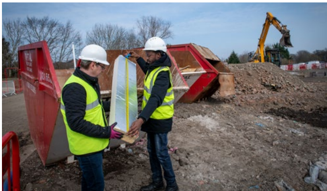
Figure 5: Measuring length of material before going into the skip
